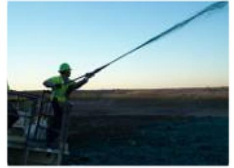
Quick Cover dries to form a uniform coating on top of the waste. Drying time is typically 30-minutes to one-hour depending on weather conditions. During windy conditions, the slurry may need to be sprayed from multiple directions to ensure proper coverage.
