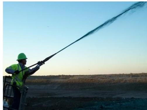
Quick Cover LT dries to form a uniform coating on top of the waste. Drying time is typically 30 minutes to one hour depending on weather conditions. During windy conditions, the slurry may need to be sprayed from multiple directions to ensure proper coverage.
